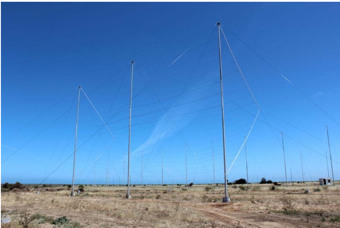
Figure 8. Buckland Park TTFD antenna construction – front antenna view.
